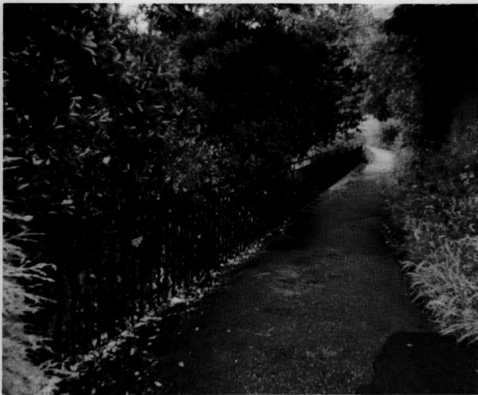
The Railings at the top of the path by St. Helena leading on to Mt. Ephraim, originally provided by the Friends in 1994, have been extended to provide protection against the steep drop on the left.
